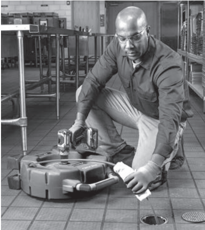
Figure 13 – Applying Lubricant to the Cable Sheath
