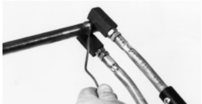
Figure 6 – Soudage du raccord
