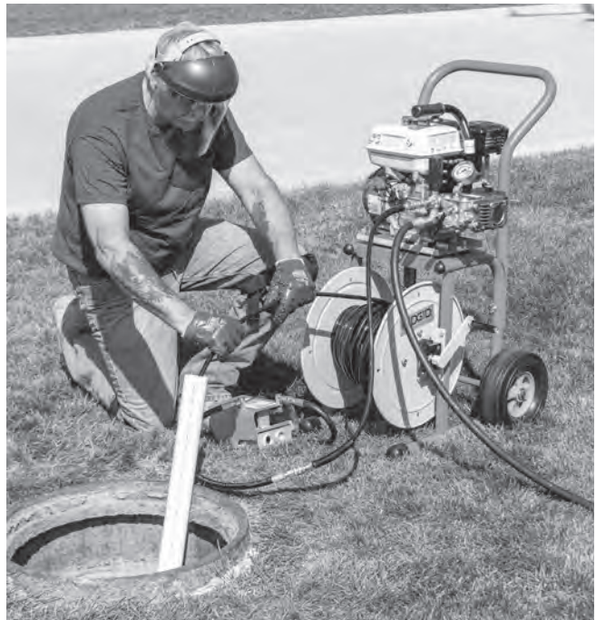
Figure 11 – Extending the Drain Opening to the Operation Point
