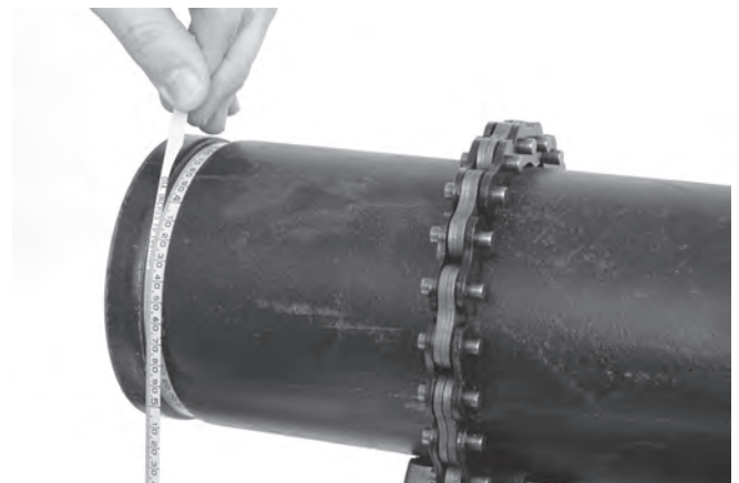
Figure 17 – Checking Groove Diameter with a Diameter Tape
