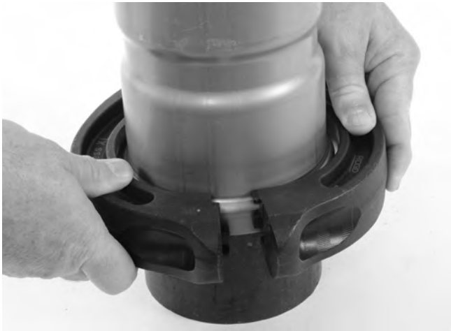
Figure 10 – Installing Press Ring Onto Fitting
