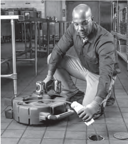
Figure 13 – Applying Lubricant to the Cable Sheath
