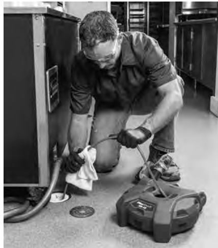
Figure 15 – Applying Lubricant to the Cable Sheath
