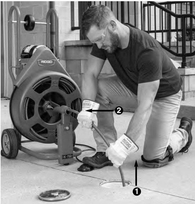
Figure 13 – (1) Pulling Cable and (2) Feeding into the Drum
