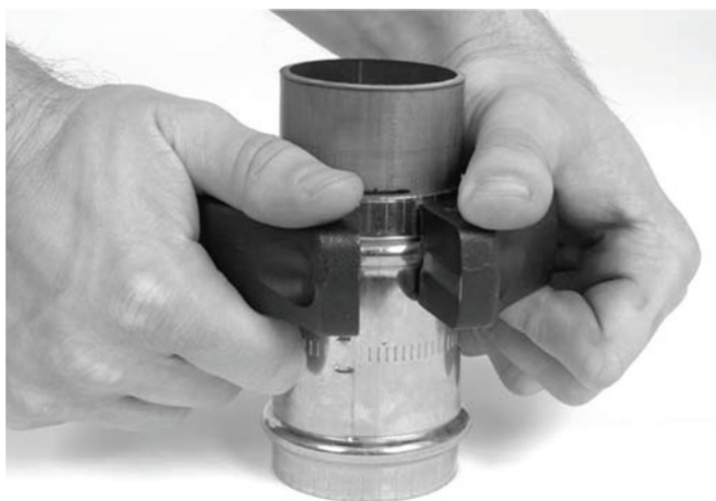
Figure 9— Installing Press Ring Onto Fitting
