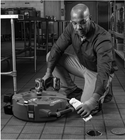
Figure 13 – Applying Lubricant to the Cable Sheath
