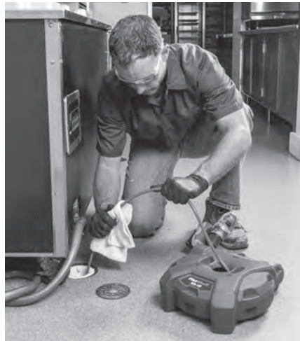
Figure 15 – Applying Lubricant to the Cable Sheath
