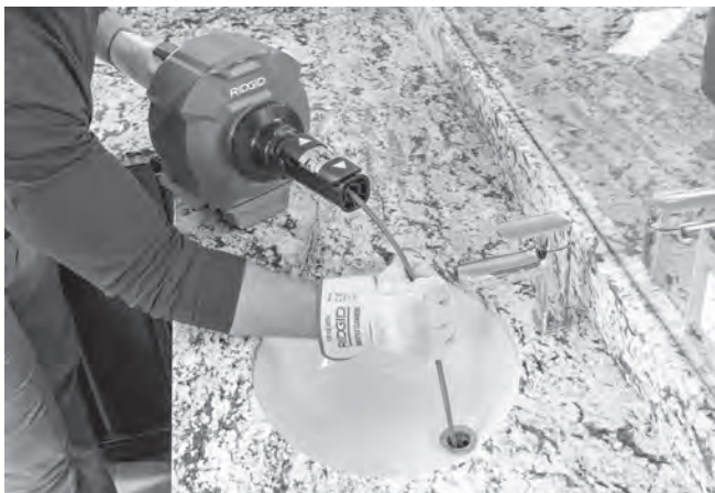
Figure 14 – Manually Feeding Cable
