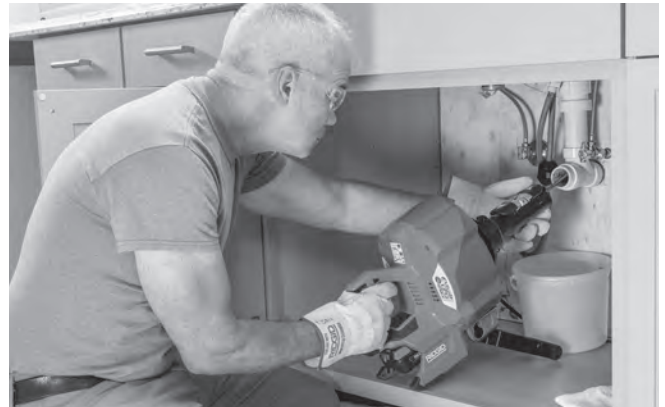
Figure 13 – Feeding Cable With AUTOFEED Unit
