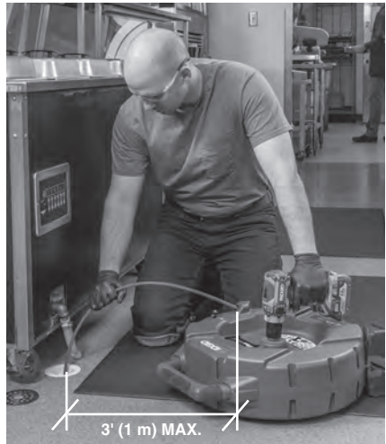
Figure 11 – In Operating Position
