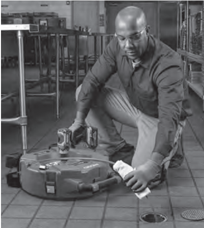
Figure 13 – Applying Lubricant to the Cable Sheath
