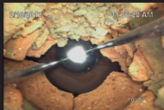
Intersection with Clay Sewer Lateral
