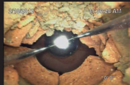
Intersection with Clay Sewer Lateral
