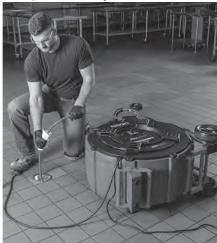
Figure 11 – Lubrification de la gaine de câble
