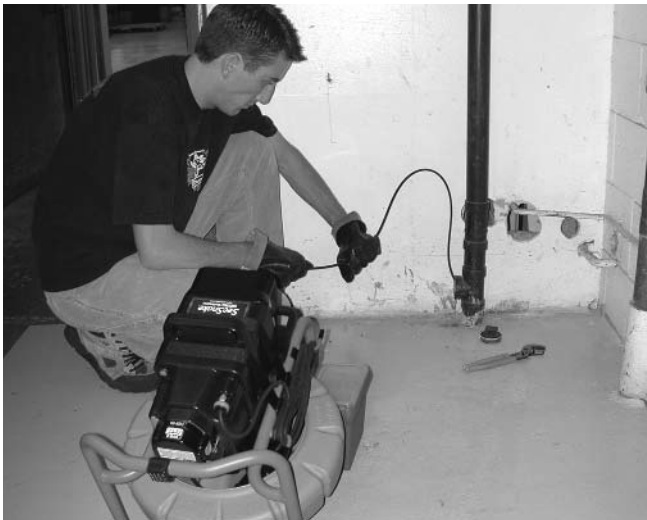
Figure 16 – Incorrect Hand Position on Push Cable
