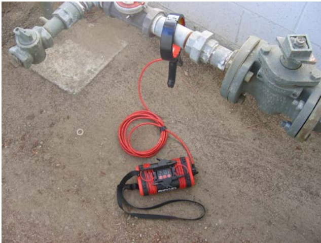
Figure 9: Inductive Clamp Attached to a Conductor
