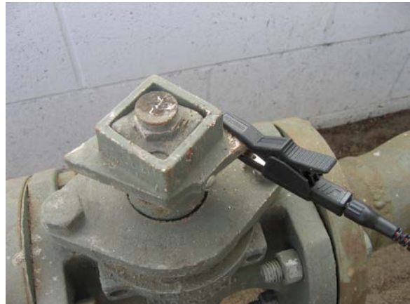
Figure 5: Connecting to a Line
