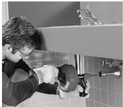
Figure 8 – Power-Spin Used By Hand
