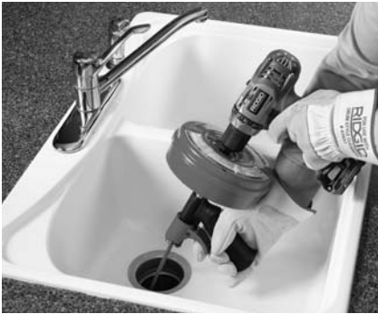
Figure 8A – Power-Spin Powered By Battery Drill
