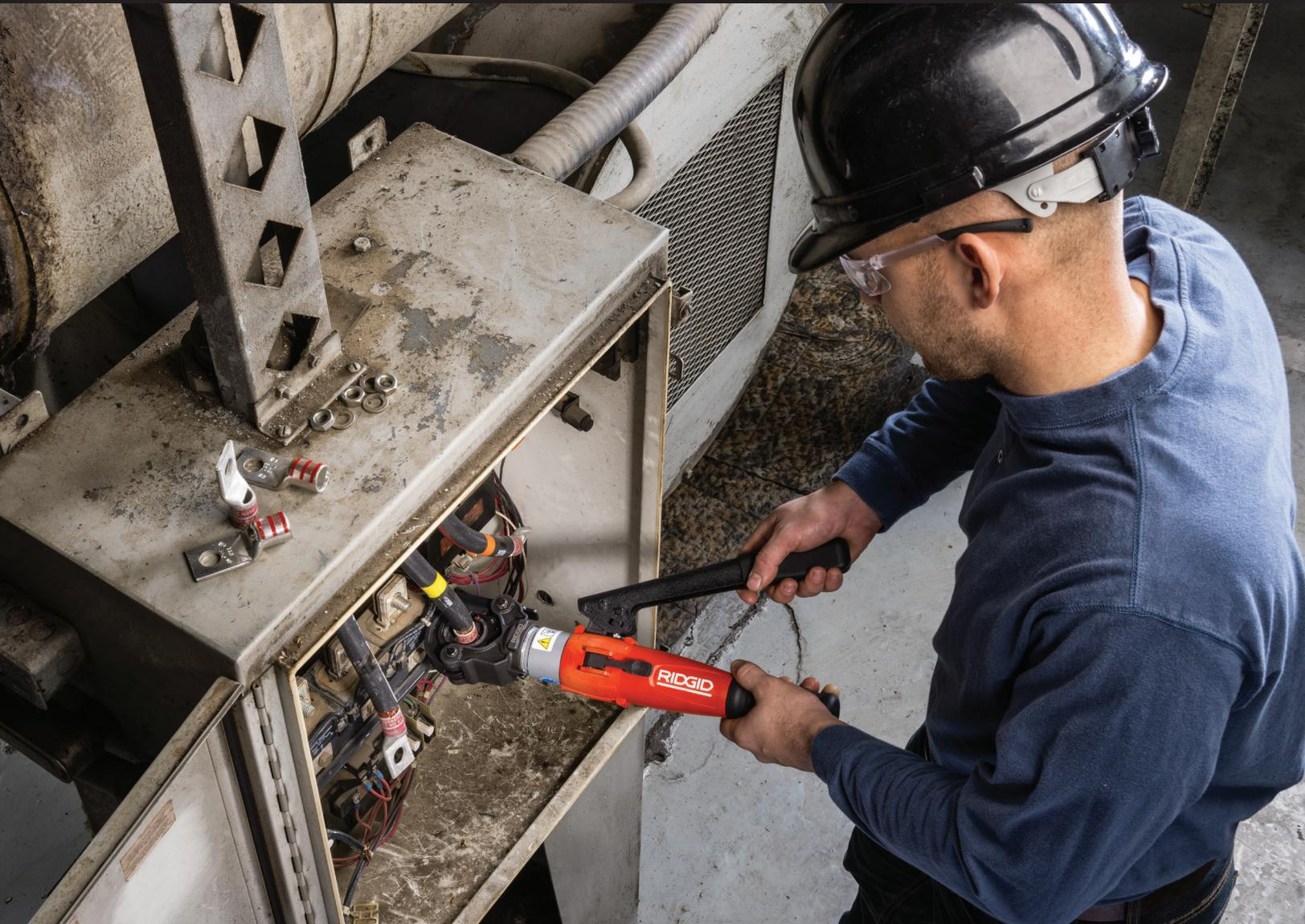
**Low handle force and RapidAdvance™ technology maximize productivity when crimping up to 600 kcmil (MCM) Copper and 350 kcmil (MCM) Aluminum.**
