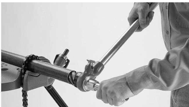
Figure 2 – Reaming End of Pipe
